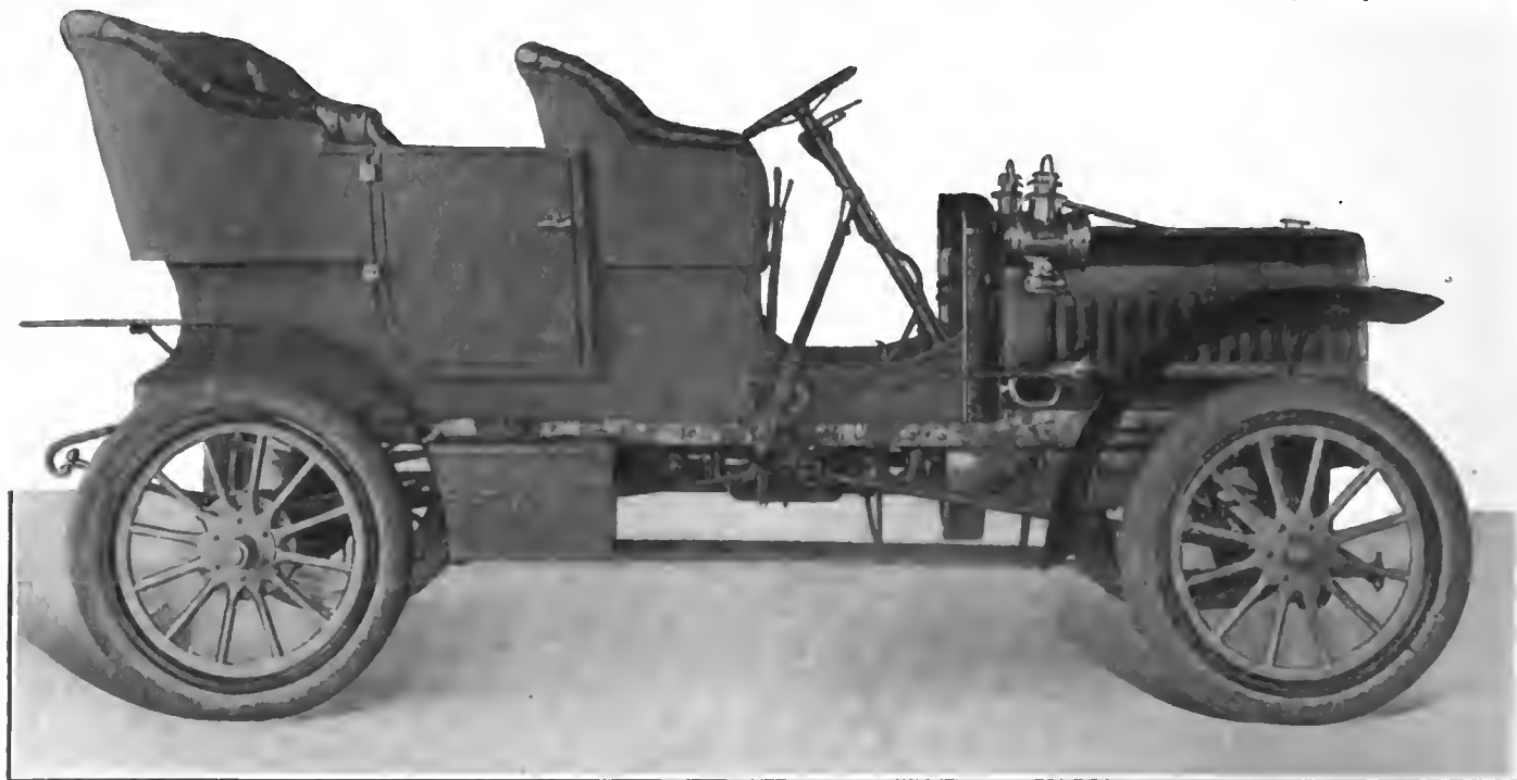
MOLINE MODEL C 18-20-HORSEPOWER, FOUR-CYLINDER LIGHT TOURING CAR FOR 1906.
